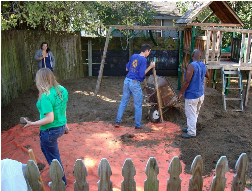
Fig. 2. Example of soil intervention using geotextile and clean soil emplacement. In hours the soil lead on the surface of the children's play area decreased from ~700 ppm to ~5 ppm. The cost was about $100 per child for this activity. Photo credit: HW Mielke, Department of Pharmacology, Tulane University School of Medicine.
